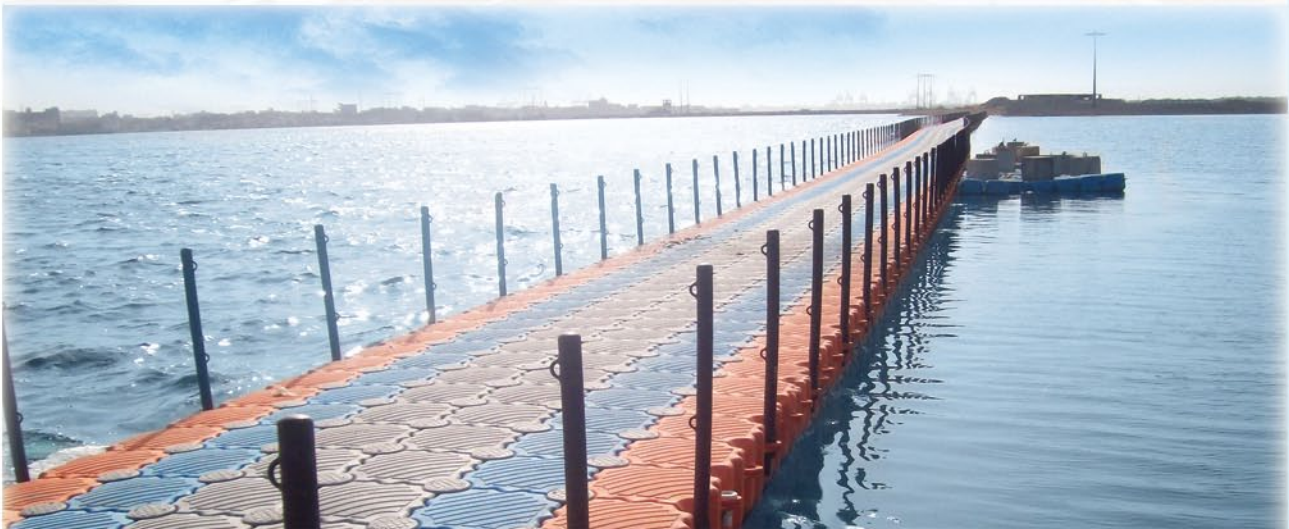
PAKISTAN'S LONGEST FLOATING BRIDGE AT SHAHEED BENAZIR BHUTTO PARK - KARACHI
