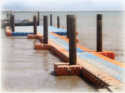
Construction of Floating Jetties and Pontoons
