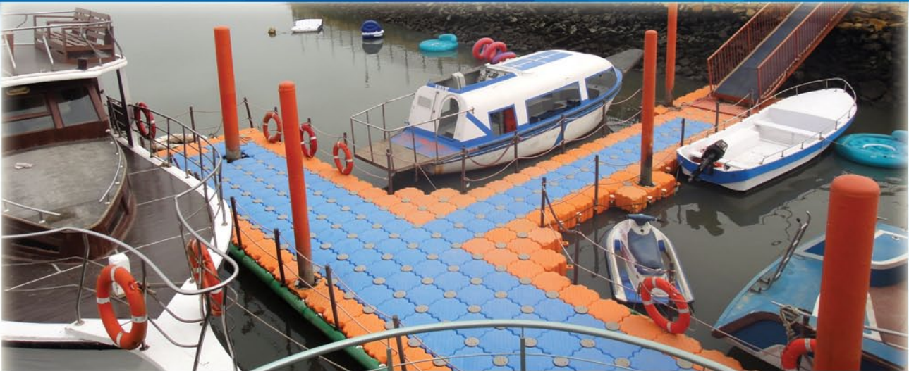
FLOATING JETTY AT SAVOR RESTAURANT - KARACHI
