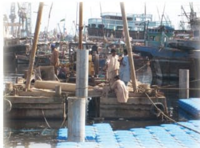
Marine Piling and Under Water Anchorage
