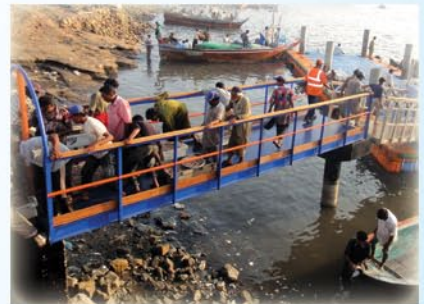
Floating, Concrete and Steel Walkways
