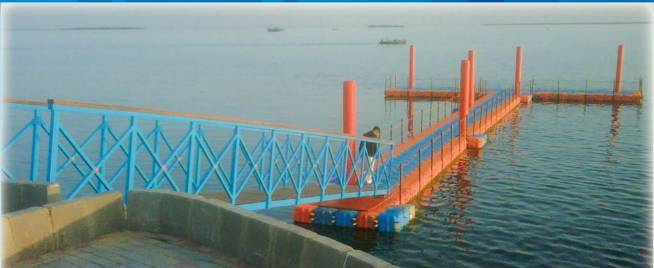
FLOATING JETTY AT AIRMEN GOLF COURSE (PAF) - KARACHI
